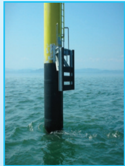
2010 - Arklow Bank Offshore Windfarm – The installed Retrowrap HD with new berthing fender
