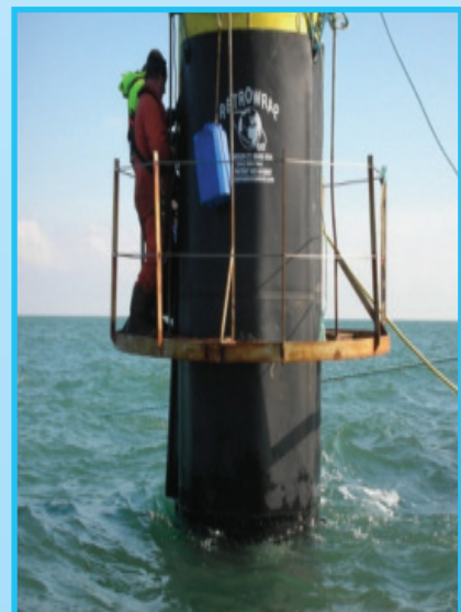
Arklow Bank Offshore Windfarm – During installation of the Retrowrap
