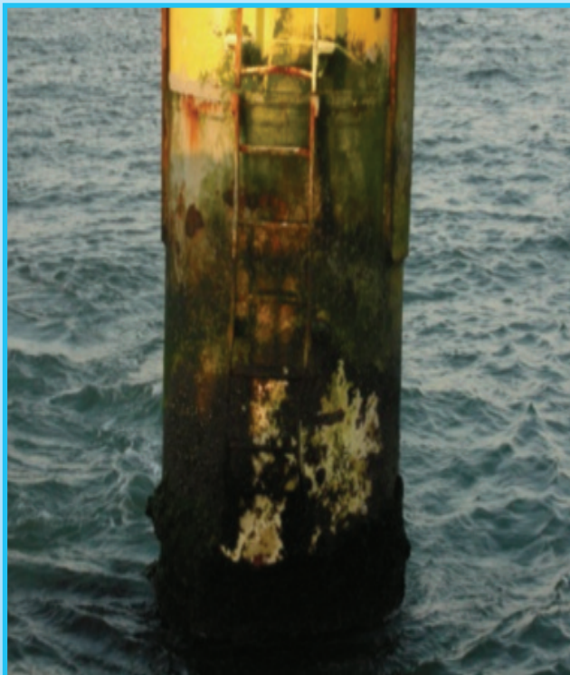
Arklow Bank Offshore Windfarm – The Corroded Met Mast Pile
