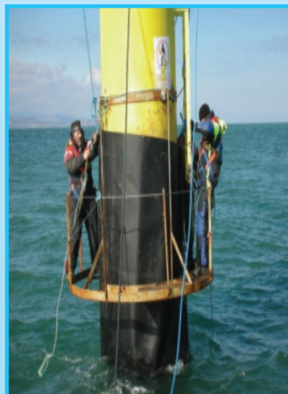
Arklow Bank Offshore Windfarm – During installation of the Retrowrap
