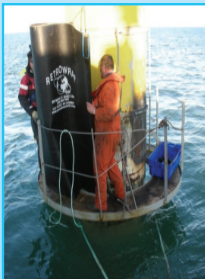
Arklow Bank Offshore Windfarm – During installation of the Retrowrap
