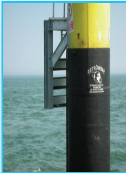
2010 - Arklow Bank Offshore Windfarm – The installed Retrowrap HD with new berthing fender
