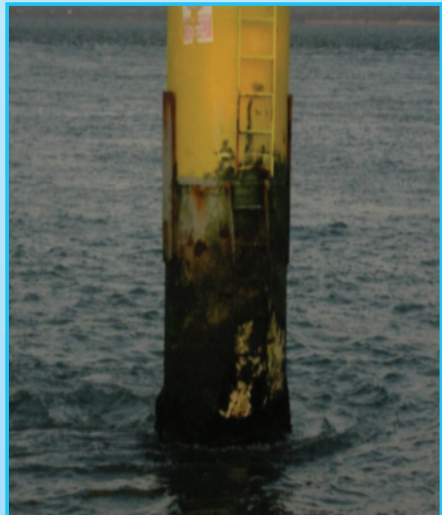
Arklow Bank Offshore Windfarm – The Corroded Met Mast Pile
