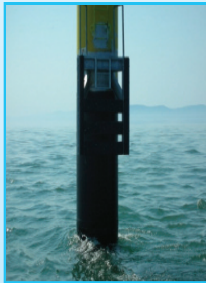
2010 - Arklow Bank Offshore Windfarm – The installed Retrowrap HD with new berthing fender
